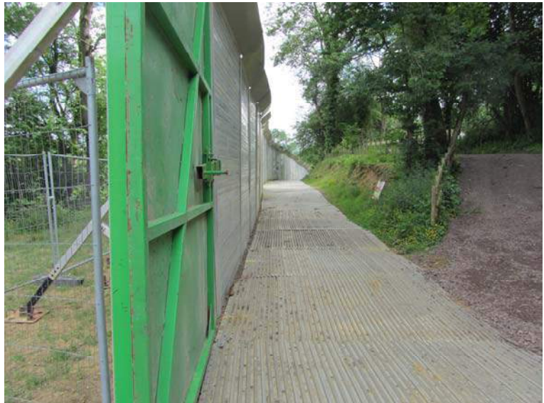
Fig. 10-5 - A custom-made fence designed to create an impregnable event perimeter. Block and mesh panels form an inner fence to create a moat in which security can operate.. Photo courtesy of The Event Safety Shop, LTD.
