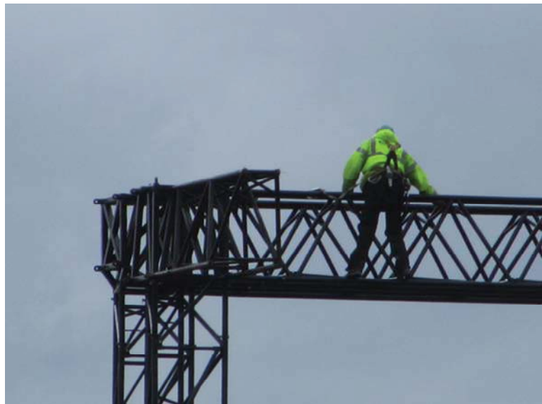
Fig. 9-2 – Example of a climber clipped in on a wet day. This is an example of appropriate fall protection. Photo courtesy of The Event Safety Shop, LTD.
