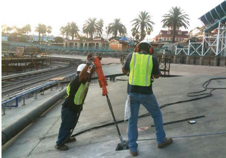
Fig. 9-1 – Installing an Earth Anchor. Earth anchors can be an effective and space efficient alternative to using bulk weight to ballast structures and rigging.
