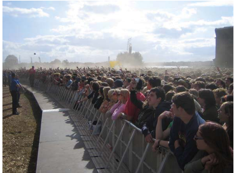
Fig. 10-6 - A standard concert stage barrier, note the diagonal bracing stays which allow the barrier to resist horizontal load. Note also the extended rear plate allowing security personnel easy access and a safe platform from which to assist or rescue the public. Photo courtesy of The Event Safety Shop, LTD.
