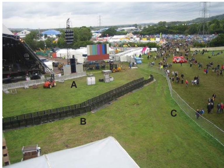
Fig. 10-2 - An example of a Primary (silver, A) and Secondary (black, B) barrier lines being installed with block-and-mesh (C) being used to delineate public and working areas. Photo courtesy of The Event Safety Shop, LTD.
