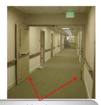
Cross corridor doors as part of smoke barrier held in place with magnetic holdopen device released by smoke detectors or fire alarm
