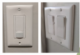
Occupant sensors, dimmers, automatic daylight sensors meet requirements
