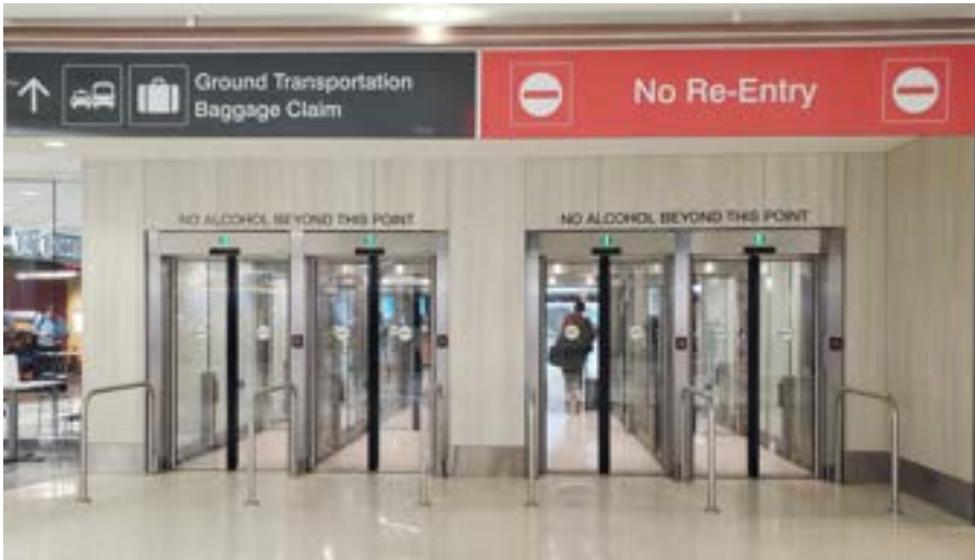
Anchorage, AK airport exit lane breach control systems.
