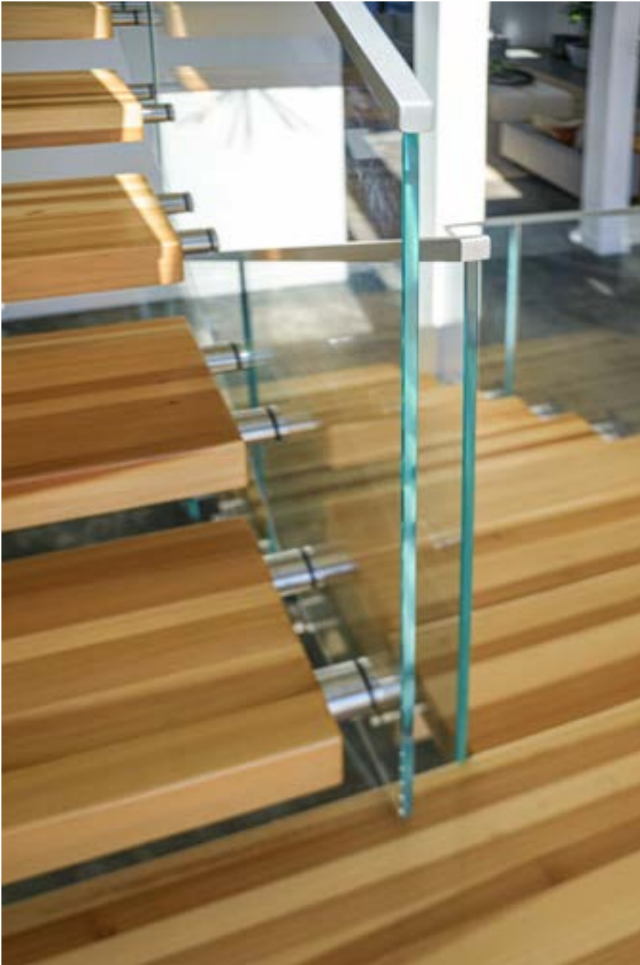
Illustration B: Shows the an open riser mono stringer stair with open ended treads.
