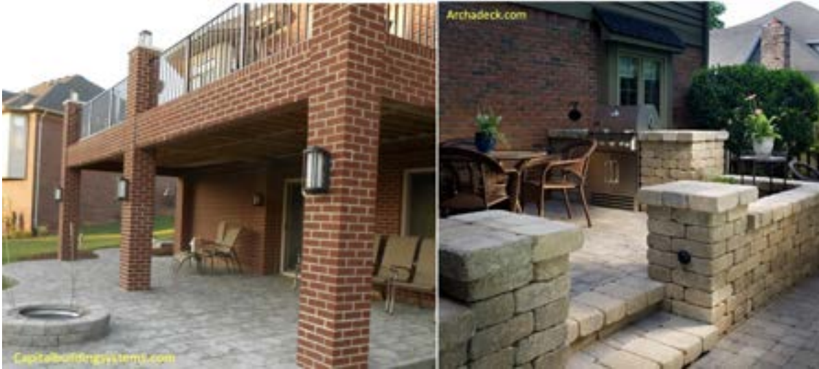
Figure 3. Unenclosed and enclosed attached accessory structure nonconforming with current requirements.
