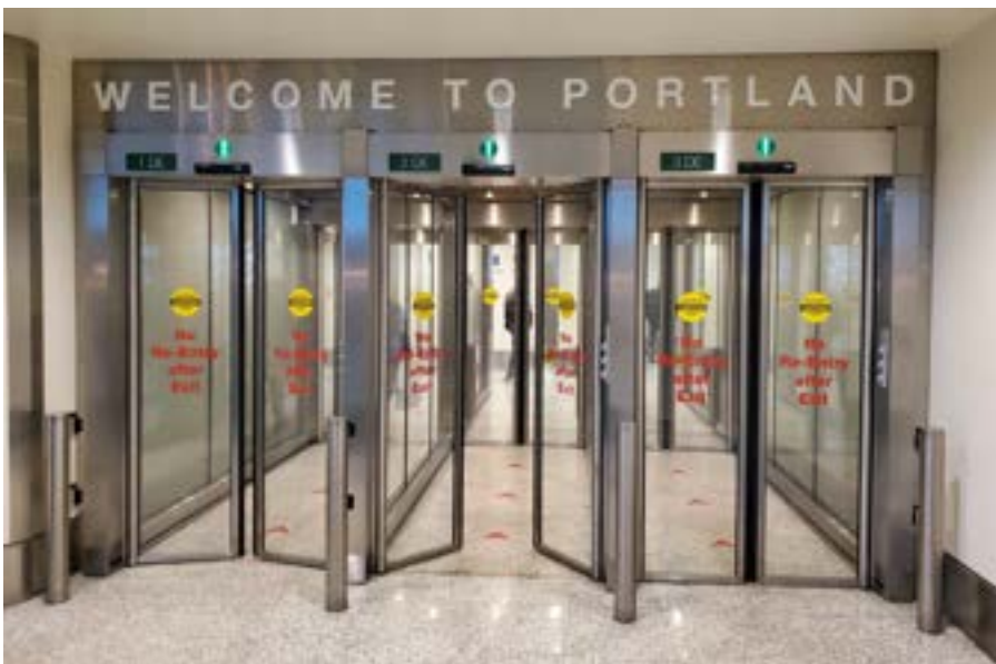
Portland, OR airport exit lane breach control systems.
