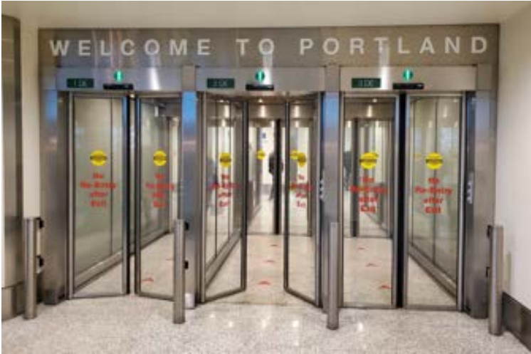
Portland, Oregon airport exit lane breach control system.
