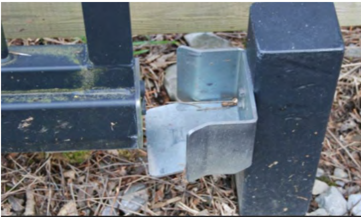
(Receiver Guide/ Gate Stop Below)
