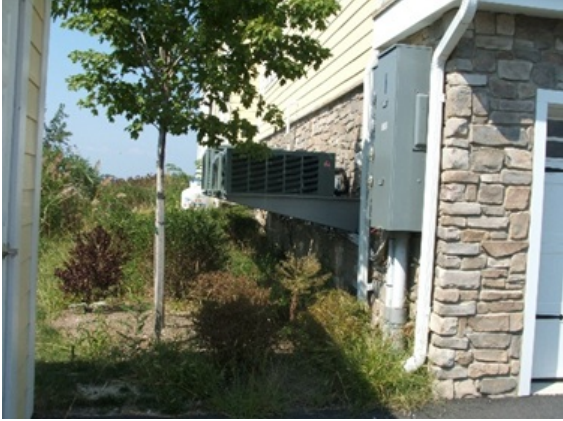
Equipment on wall mounted platform
