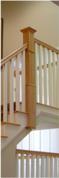
Handrail to Post as permitted by code
