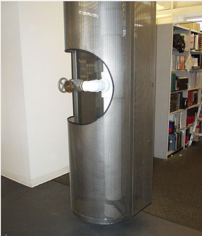
Example of a cowl. Concern with access for fire department and operation.
