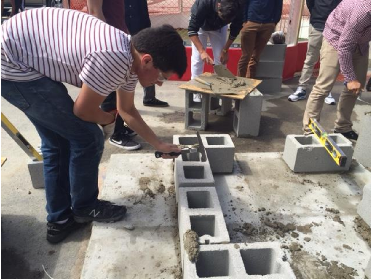
An ECTA student laying blocks.
