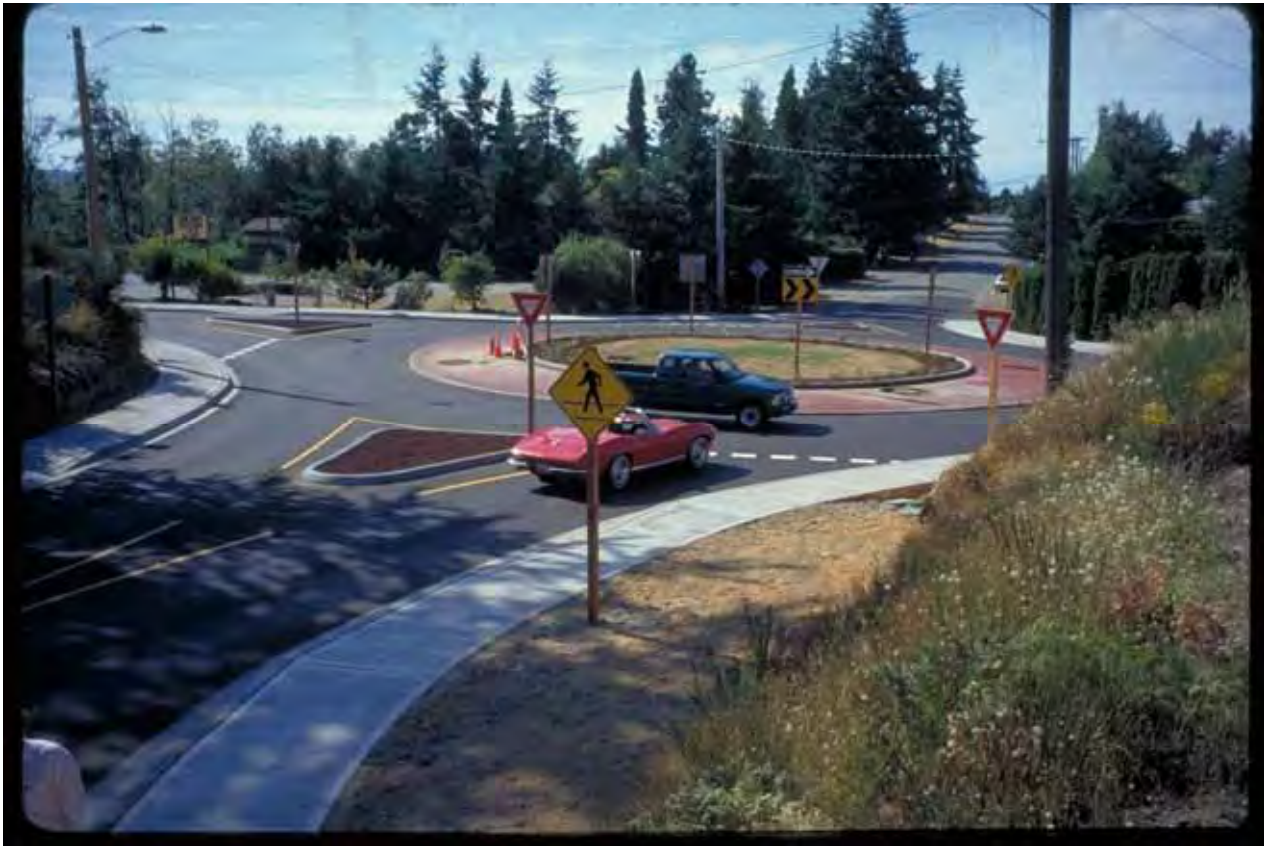
A typical modern roundabout in University Place, WA. At the roundabout entry, the clear width provided is only approximately 13 feet: this is an intentional design element to keep vehicle speeds low. Photo: IMG0032.jpg
