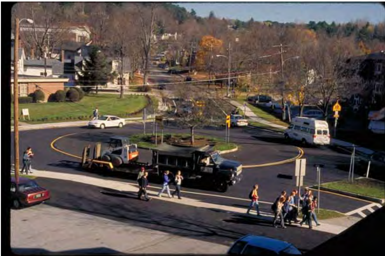
A typical modern roundabout in University Place, WA. At the roundabout entry, the clear width provided is only approximately 13 feet: this is an intentional design element to keep vehicle speeds low. Photo: IMG0032.jpg
