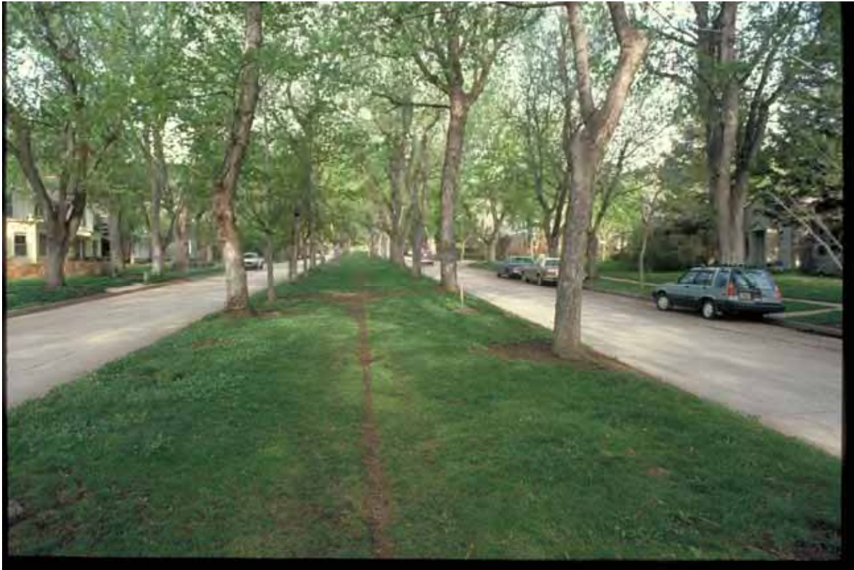
An example of a roadway with a raised median and approximately 17 feet of clear width on each side of the median. Photo: median.jpg
