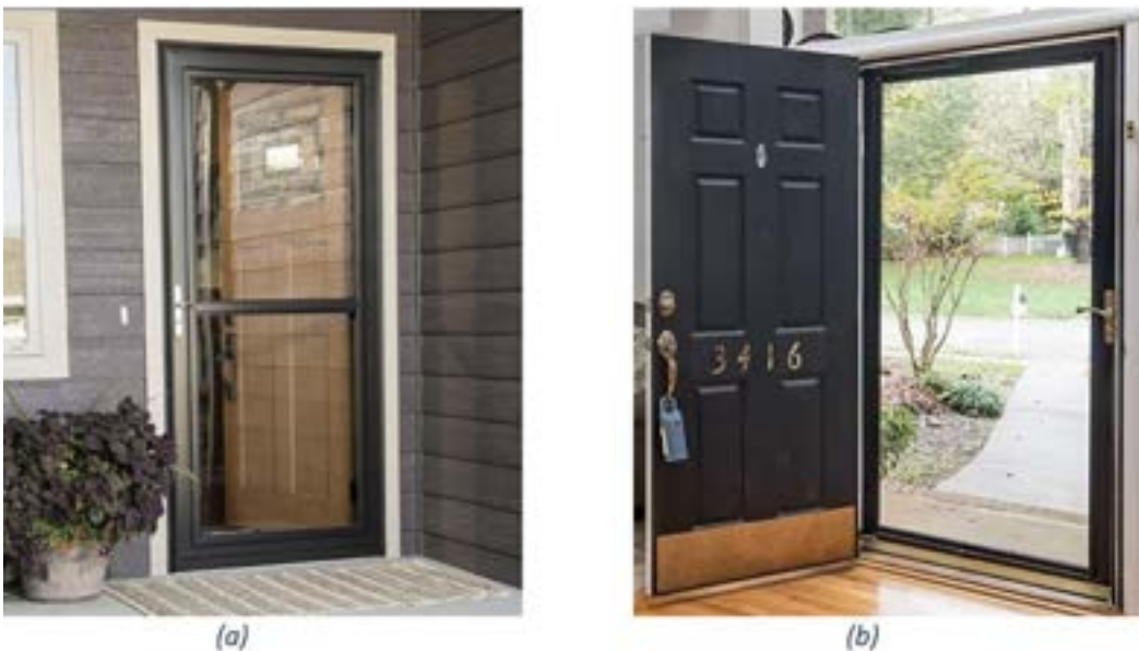
Figure 2. Protection for exterior doors (a) storm door, (b) kickplate.
