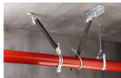
Types of piping hangars and supports
