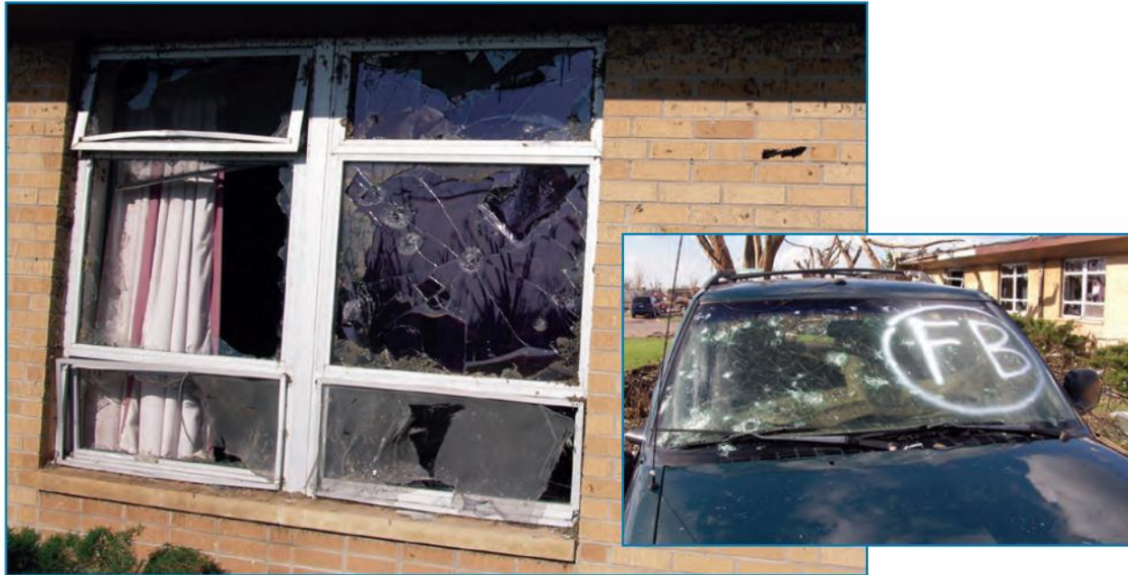
Figure 3 - Glazing damage at a hospital in Greensburg Kansas following a tornado in 2007. The craters shown in the right center pane and at the vehicle windshield were caused by the large aggregate blown from the ballasted single-ply membranes (FEMA 2012).
