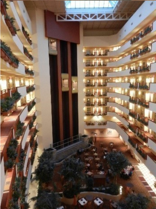
Example of elevator hoistways that are not in rated enclosures.
