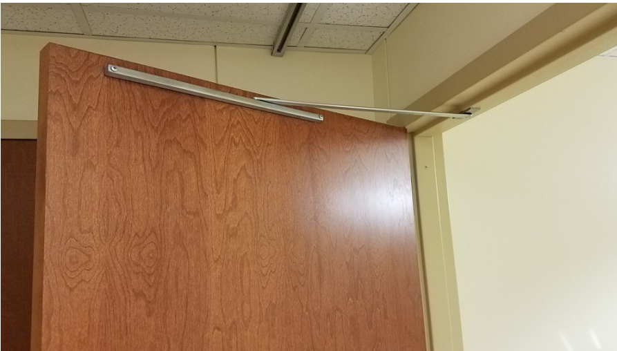
Overhead door stop.
