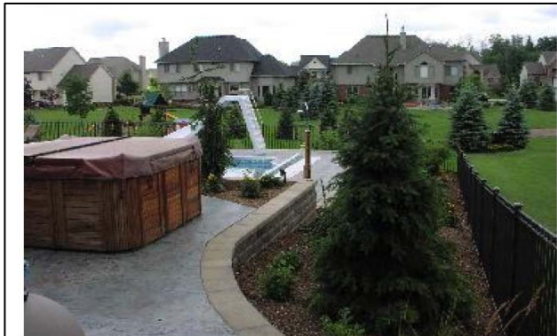
This picture illustrates two issues that arise with the current language on guards. First, we have a walking surface that is more than 30 inches above a point within 36 inches of the open side of the walking surface. Therefore a guard 36 inches high is required. Then we have adjacent fixed seating in the form of the seating around the edge of the hot tub. The seating is 42 inches above the walking surface. Therefore the total height of the guard at this location will be 78 inches. The IRC requires that the guard be able to resist a "single concentrated load (of 200 pounds) applied in any direction along the top." This will require some very substantial mounting hardware to attach the guard to the patio to resist such forces.
