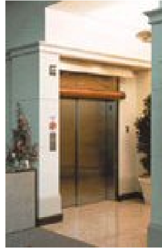
Figure 1 - Roll down barrier deploying over an elevator door (courtesy Smoke Guard)
