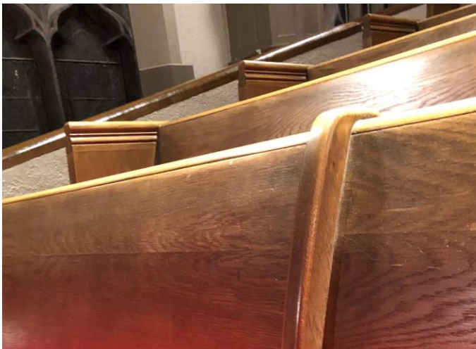
Figure 5 First United Methodist Church in Kalamazoo, Michigan Graspable end portion of a church pew Adjacent to a stepped aisle having seating on one side.
