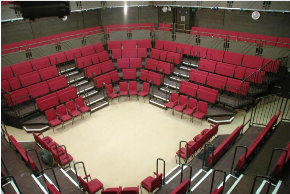
Figure 4 – U handrail on both sides of aisle.
