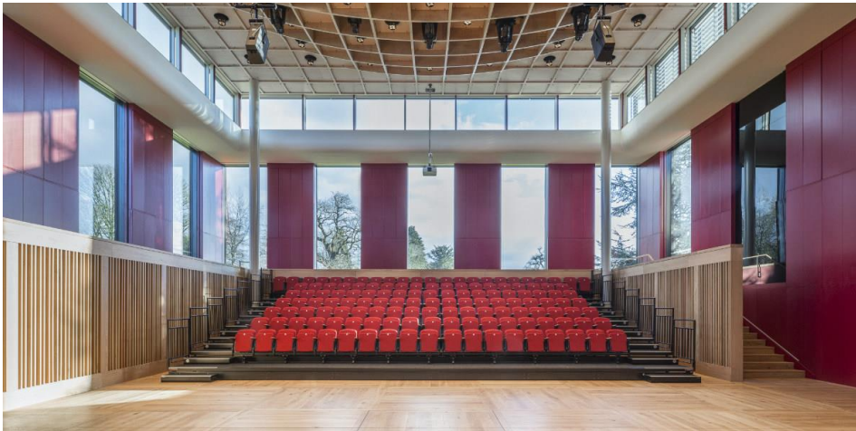
Figure 5 – guard with graspable top rails
