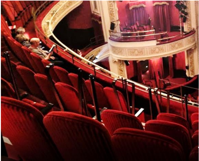
Figure 4 Royal Alexandra Theater in Toronto, Canada Mid-aisle handrail with additional knob style handrail adjacent to seats.
