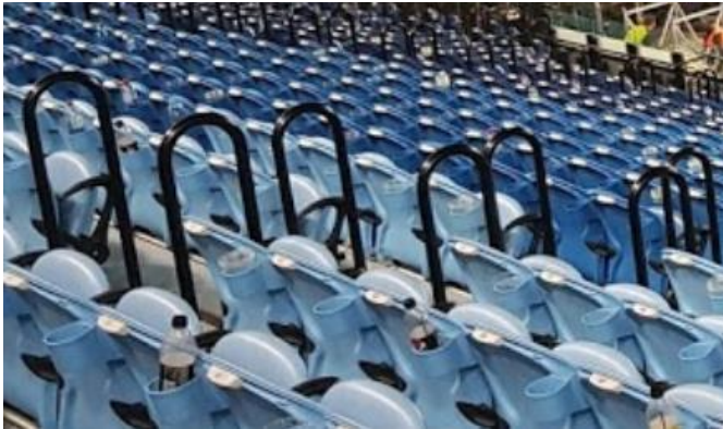
Figure 2 Rod Laver Arena in Melbourne, Australia Handrail adjacent to seats on both sides of the aisle without mid-aisle handrail.
