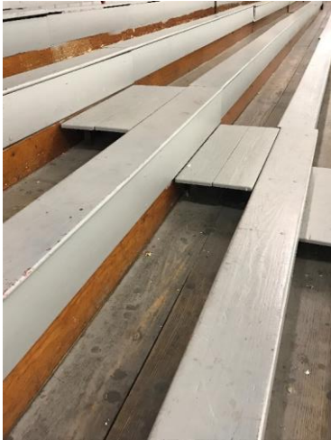
48" wide steps are inserted into the foot area and handrails are secured
