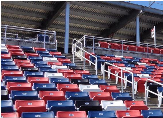
Figure 8 NASCAR Grandstand with mid-aisle handrail transitioning to handrails on each side where there are seats on neither side.
