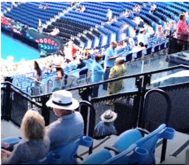
Figure 3 Rod Laver Arena in Melbourne, Australia Handrail adjacent to seats on one side of an aisle.
