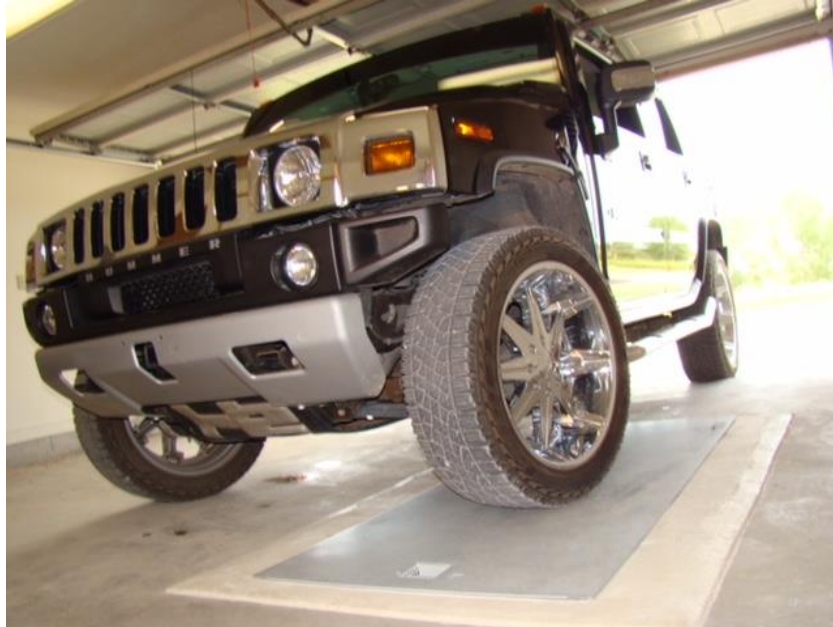
Wheel load on an operable opening to an underground storm shelter
