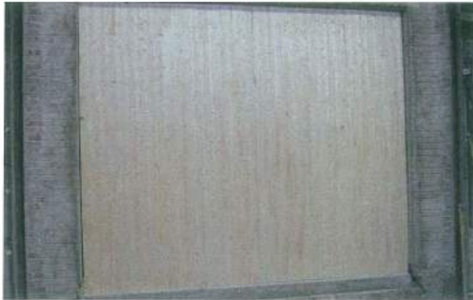
Exposed Side – CLT Wall Construction
